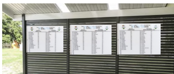
Above: Gazebo design and example of the panels to be installed displaying names of the people believed to be interred on site.
